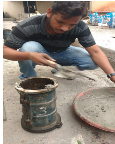
Fig. 4. Casting of cubes and cylinders
