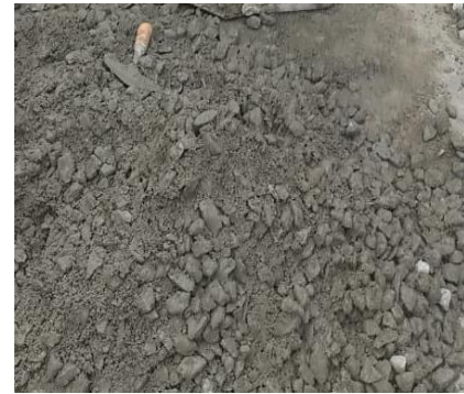
Fig. 1. Hybrid fiber reinforced concrete
