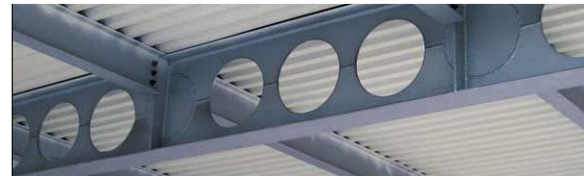
Fig. 1. Castellated beam with web opening
