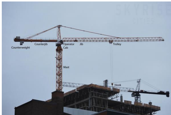
Fig. 2. Tower Crane Anatomy
