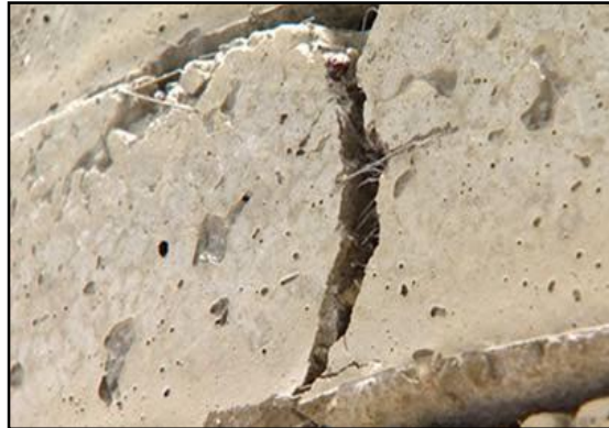
Fig. 10. Cracks formed in beam due to flexural strength test (shows fibre bonding)
