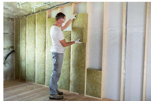
Fig. 5. Installation of thermal insulation in walls
