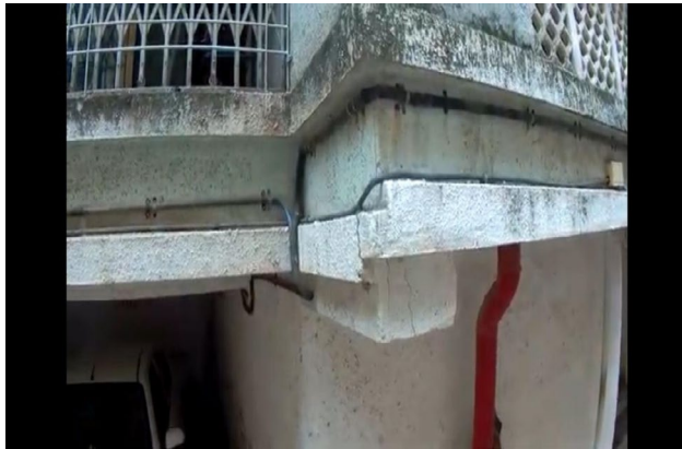
Fig. 1. Drone image of slab surface used for ImageJ analysis
