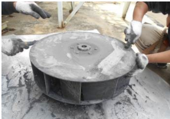
Fig. 5b. Cleaning impeller
