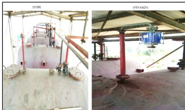
Fig. 5. Before and after implementation of solution: Breather located
