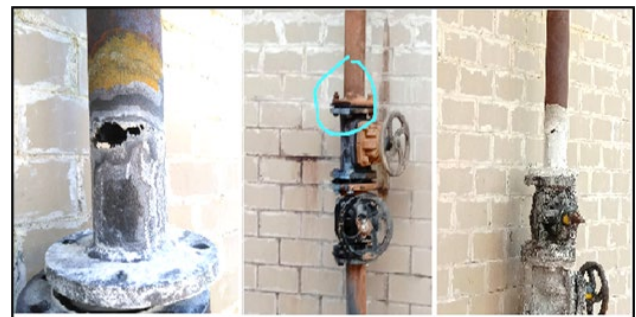
Fig. 4. Leakage points of pipe line
