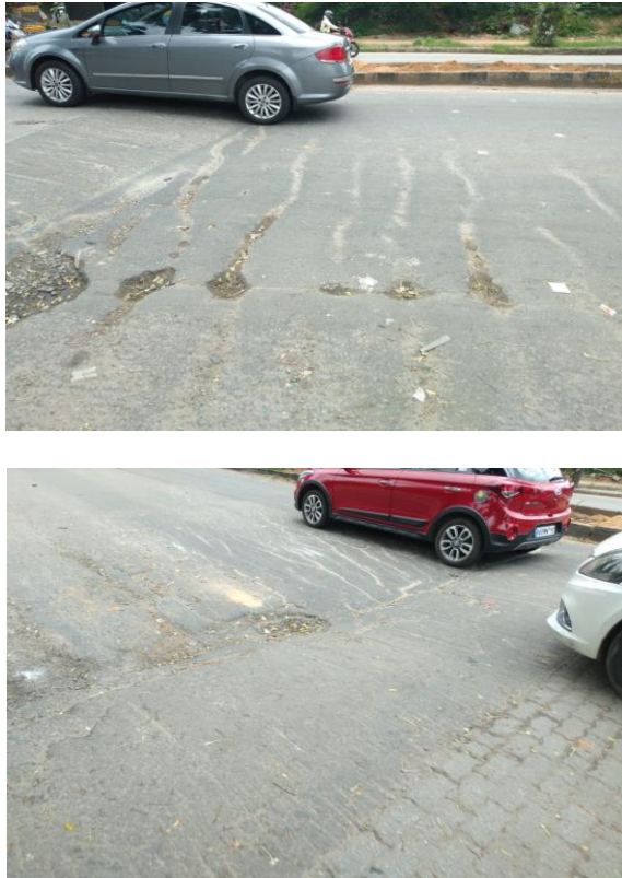
Fig. 5. Road condition in corridor
