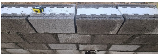
Fig. 2. External wall made of thermal blocks under construction
