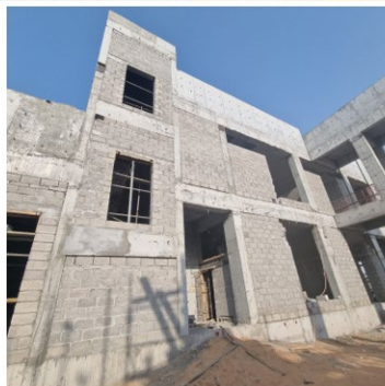
Fig. 22. External walls under construction
