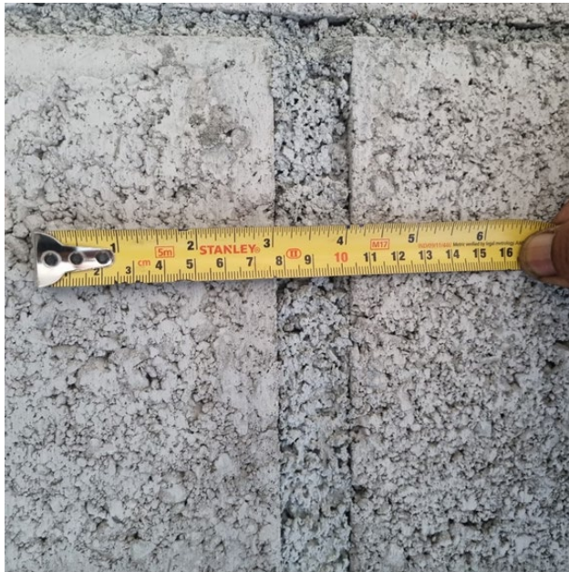
Fig. 21. Thickness of mortar joints
