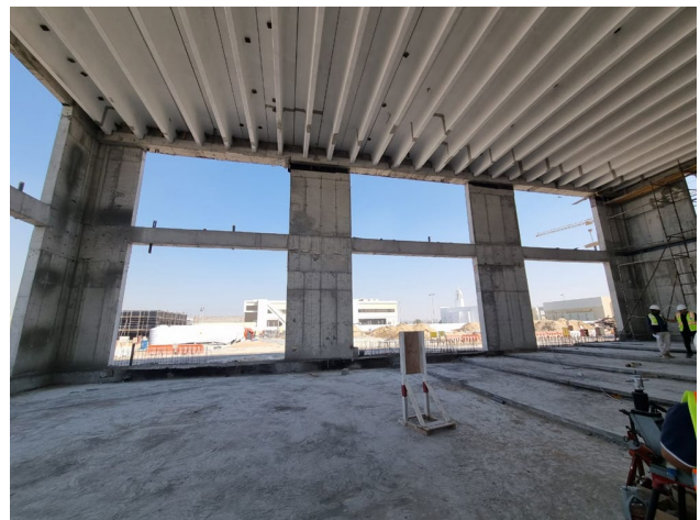
Fig. 13. Concrete frame within the external wall
