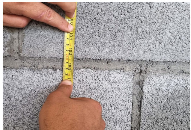
Fig. 3. Thickness of horizontal mortar joints
