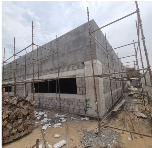
Fig. 18. Photos of external wall during construction
