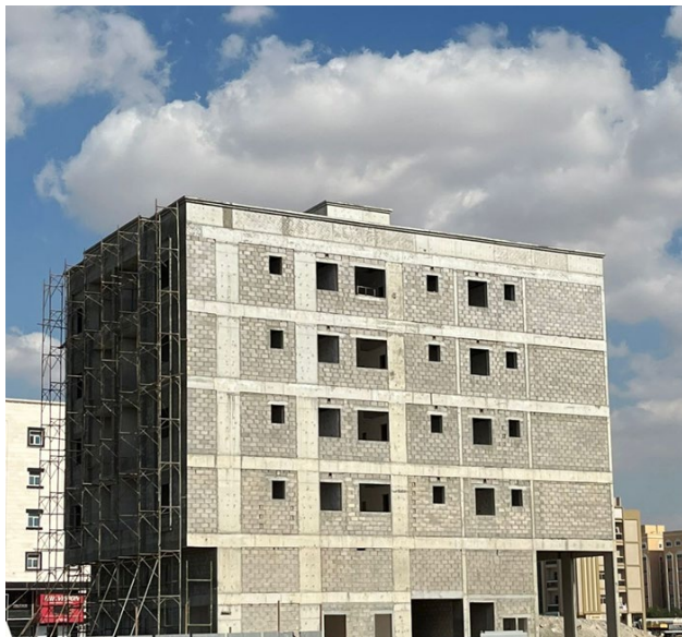
Fig. 10. External wall beams and columns
