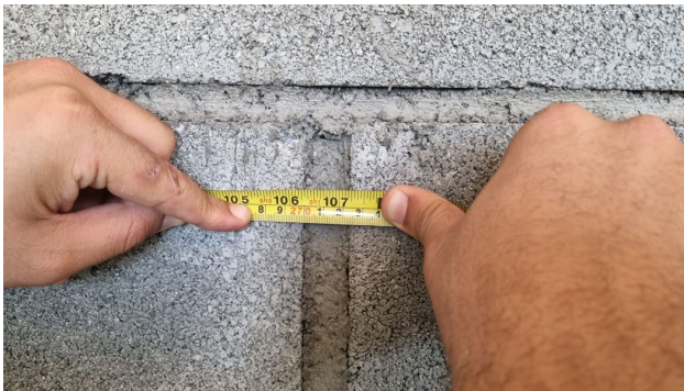
Fig. 4. Thickness of vertical mortar joints
