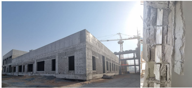
Fig. 20. External wall under construction showing external surfaces and morphology
