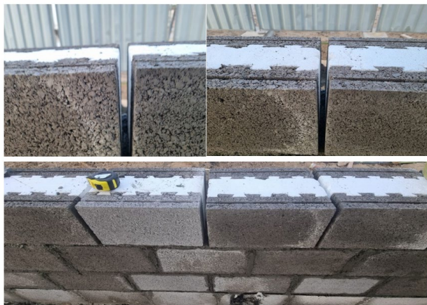
Fig. 1. Mortar joints of thermal blocks
