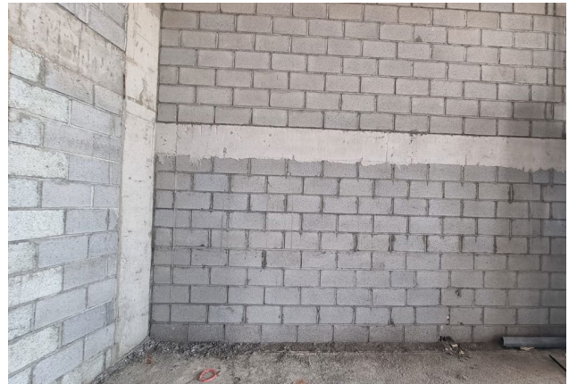
Fig. 11. Concrete stiffener beam for wall reinforcement
