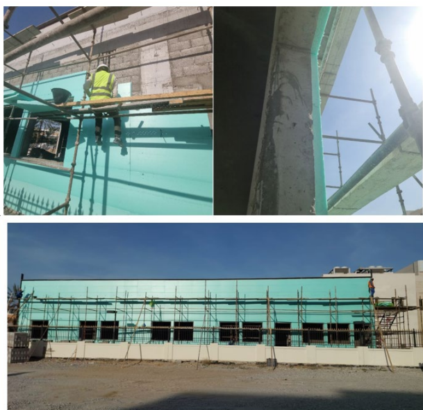
Fig. 24. Installation of insulation layer
