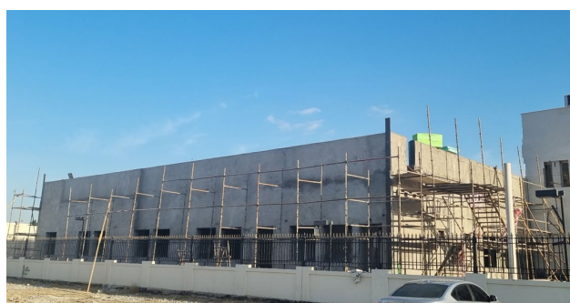
Fig. 25. Thermocoat fully applied on the external wall
