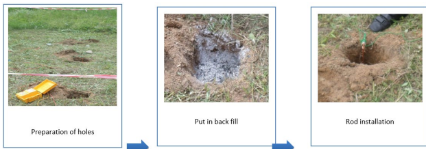
Fig. 4. Installation process for the grounding system
