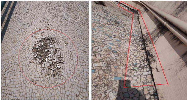
Fig. 2. China mosaic surface is found to be de bonded and Cracks on drip mould
