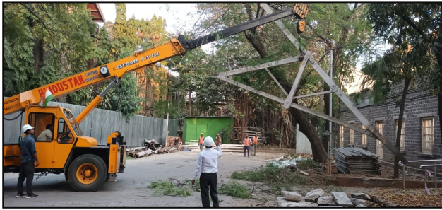
Fig. 2. Dismantling of roof with help of crane
