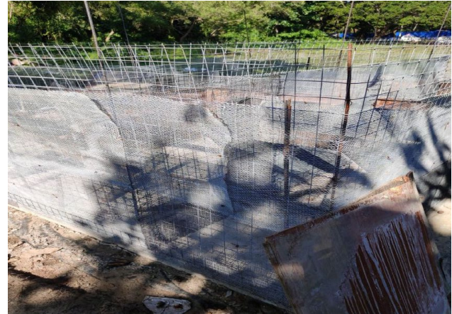
Fig. 1. Construction of bottom model
