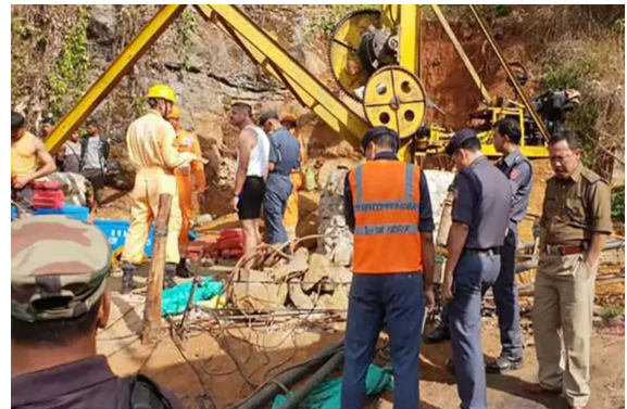
Fig. 2. Drilling of borehole for information and communication
