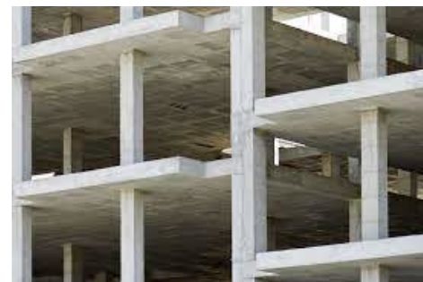
Fig. 2. Flat slab without drop panels
