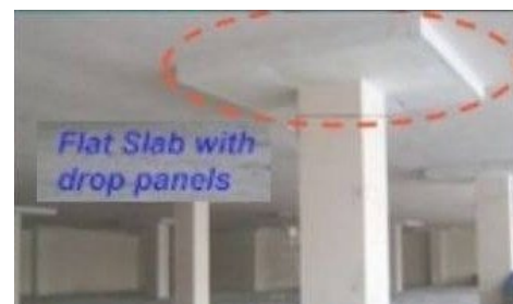
Fig. 1. Flat slab with drop panels
