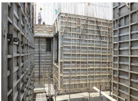
Fig. 9. Construction using mivan technology
