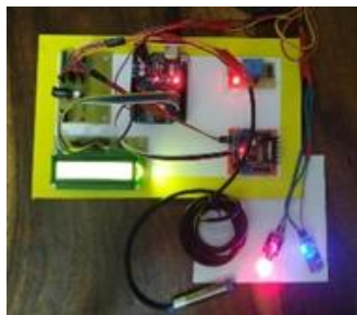
Control Panel (Electronic Components)
