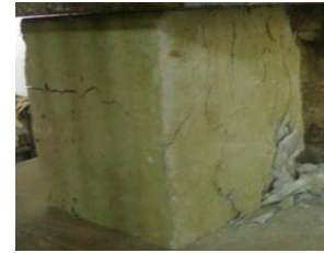
Fig. 4. Control concrete cube failure
