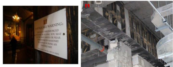
Fig. 7. Carbon fiber wrap of a beam
