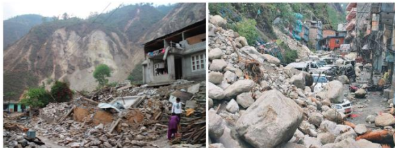
Fig. 10. Damages due to landslide
