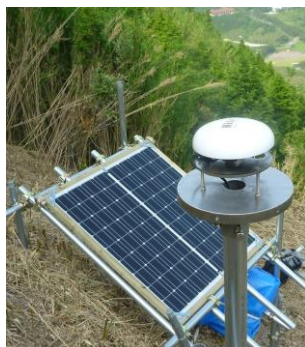
Fig. 11. GNSS reference station
