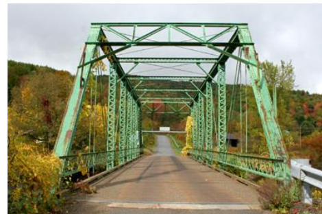
Fig. 1. Boyer Bridge, Pennsylvania
