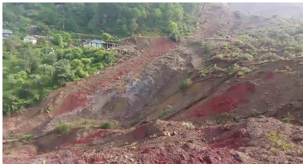
Fig. 3. Landslide in Padhar
